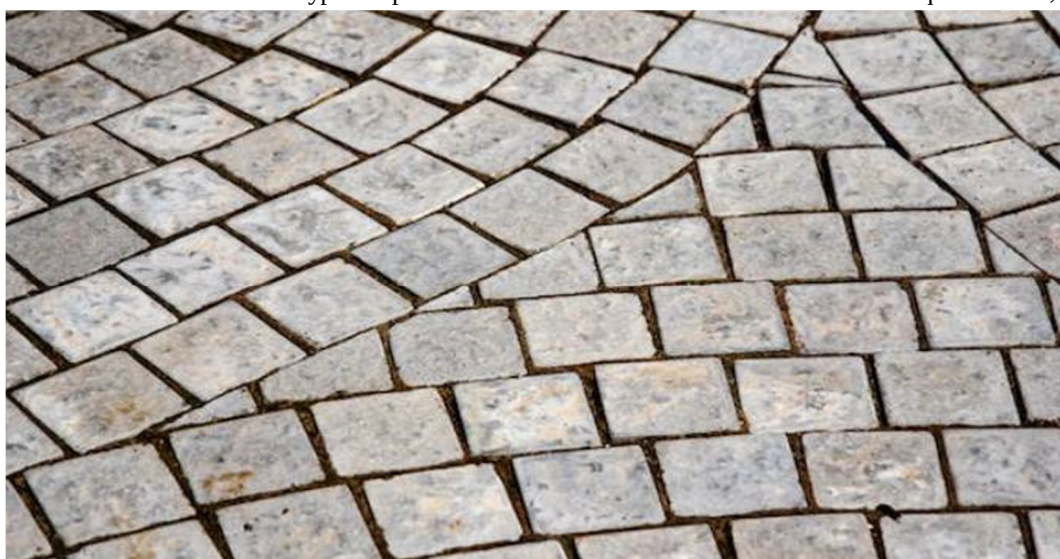
Figure 1.1: Picture Showing Paver Pavement
