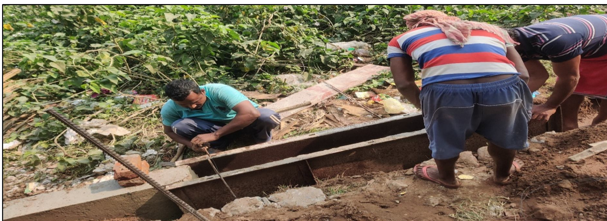
Figure 1.6: Construction of Guard Wall
