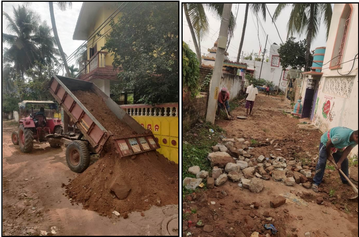
Figure 1.5: Dressing and Earthwork
