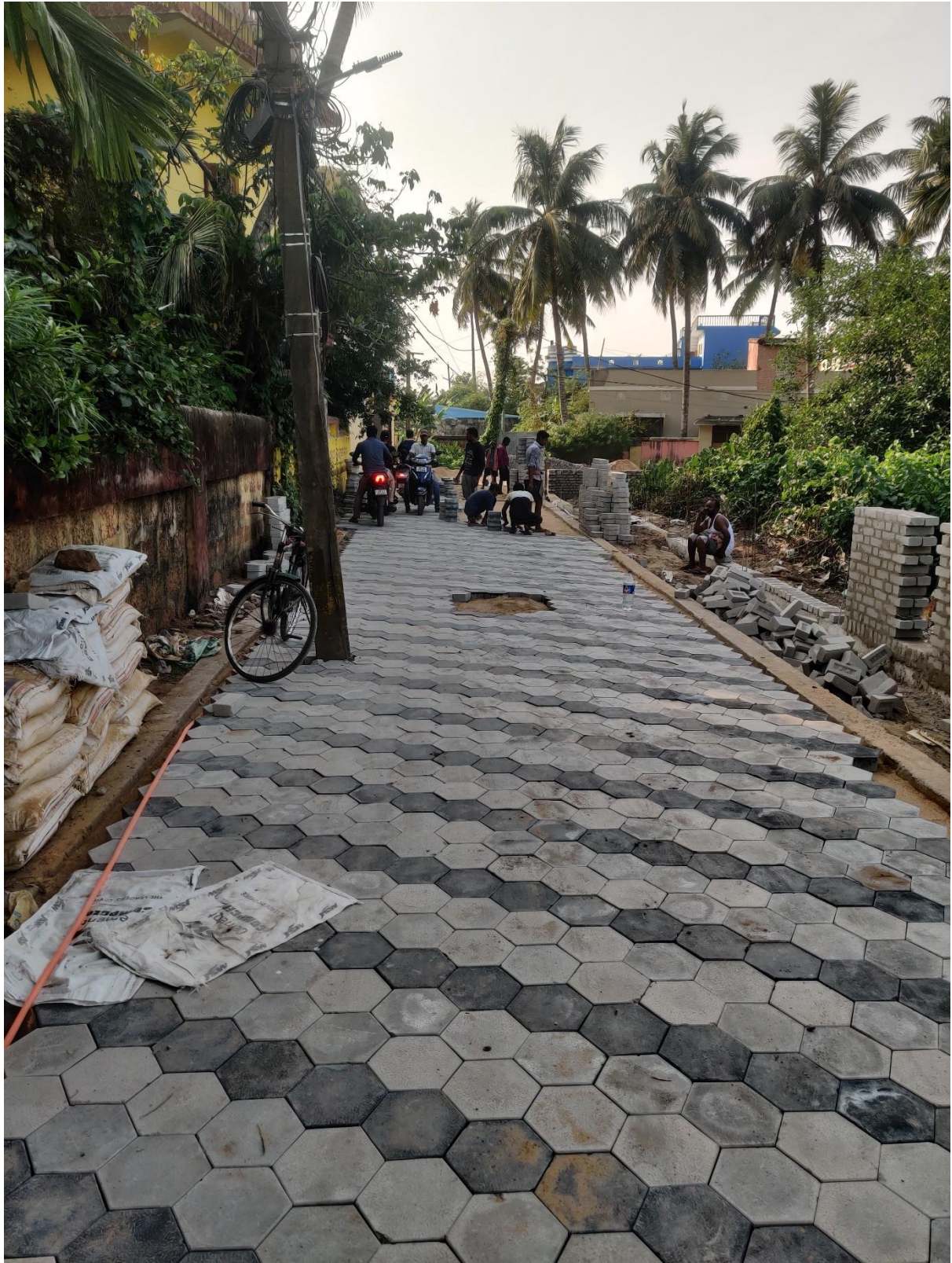
Figure 2.0: FINAL CEMENT CONCRETE PAVEMENT USING PAVER BLOCKS
