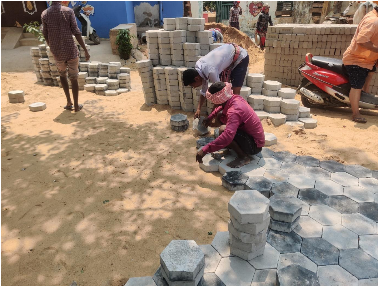
Figure 1.9: Laying of the Paver Blocks
