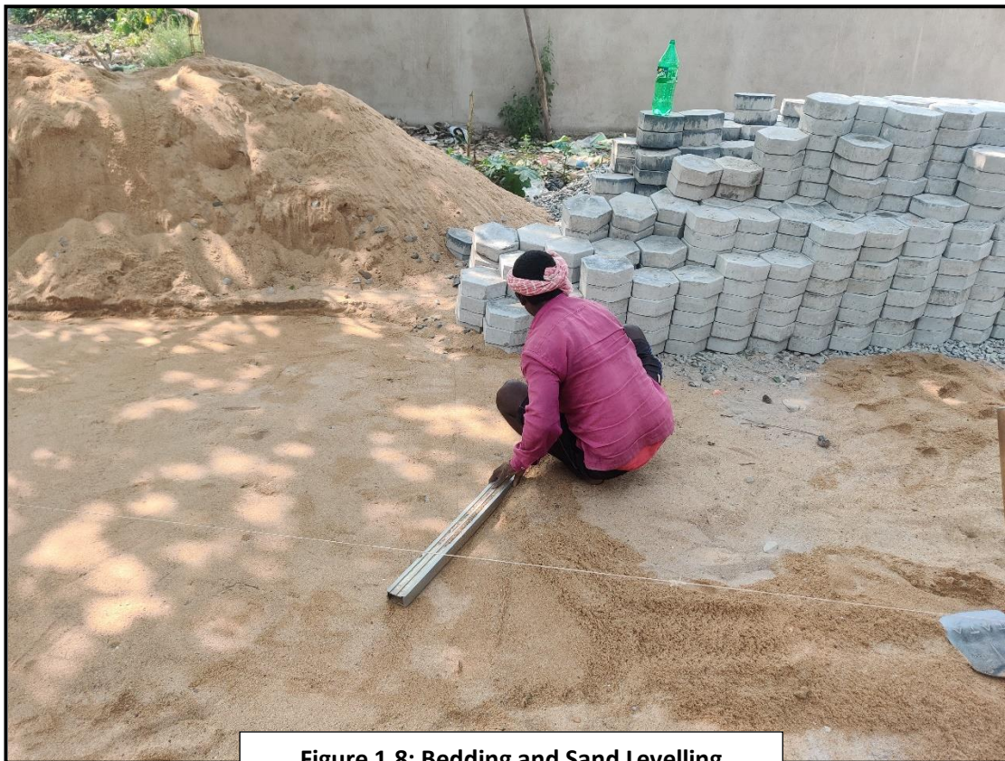
Figure 1.8: Bedding and Sand Levelling
